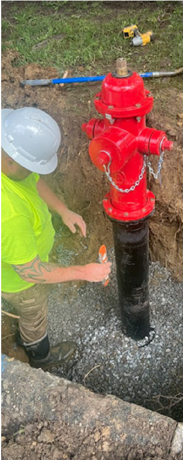
Recent fire hydrant replacement project.
